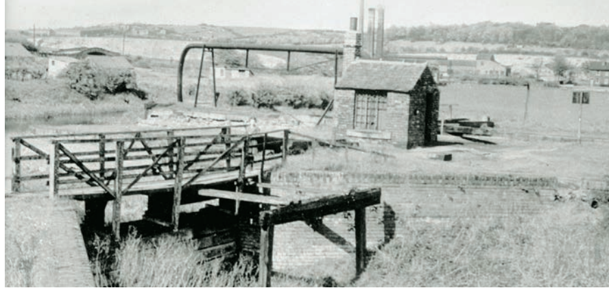
1 JUNCTION OF the Worsbrough Branch and the Dearne and Dove. Lock 18 of the Dove and Dearne canal can just be seen behind the pump house and the Worsbrough Branch is to the left of the photograph.
